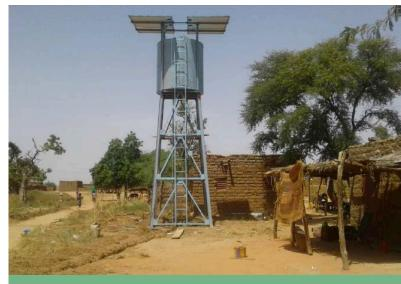
The Water tower with the solar power plant above
