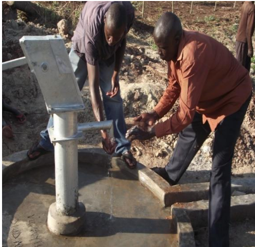
Final testing of borehole and pump
