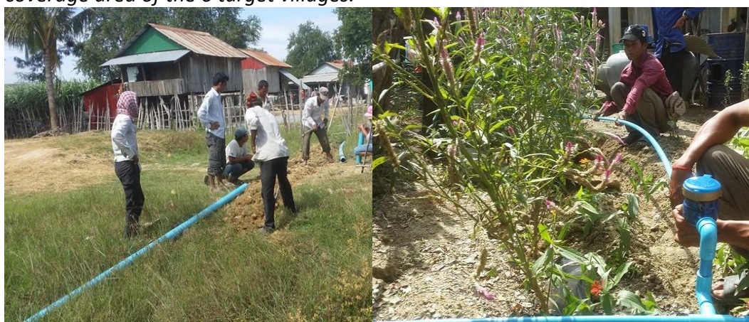
Connecting water pipes to the villages
