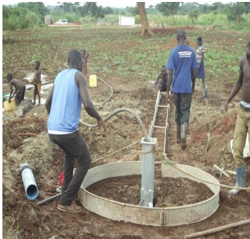
Construction of borehole
