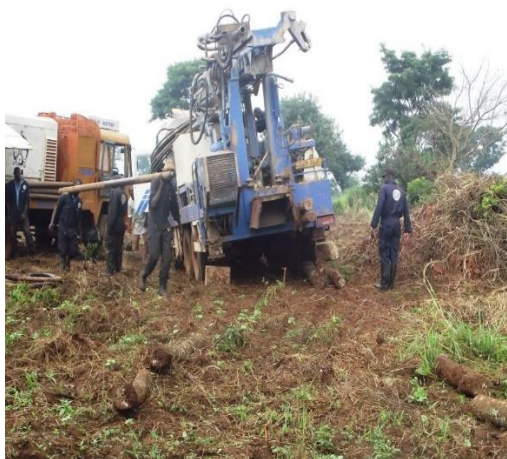
Preparation for drilling
