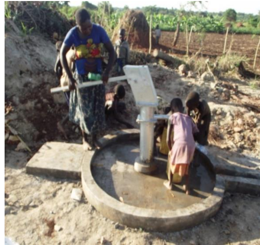
Borehole and pump in use by beneficiaries
