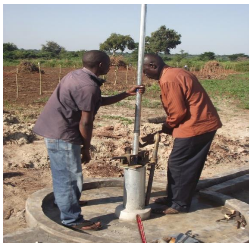
Installation of pump
