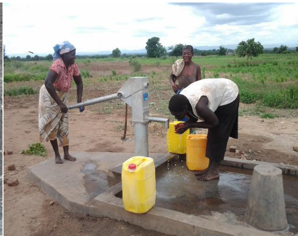
One of the five new boreholes constructed in Mlolo
