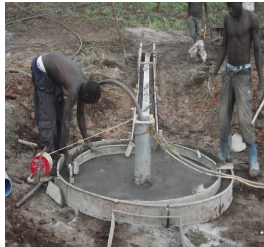
Borehole nearing completion
