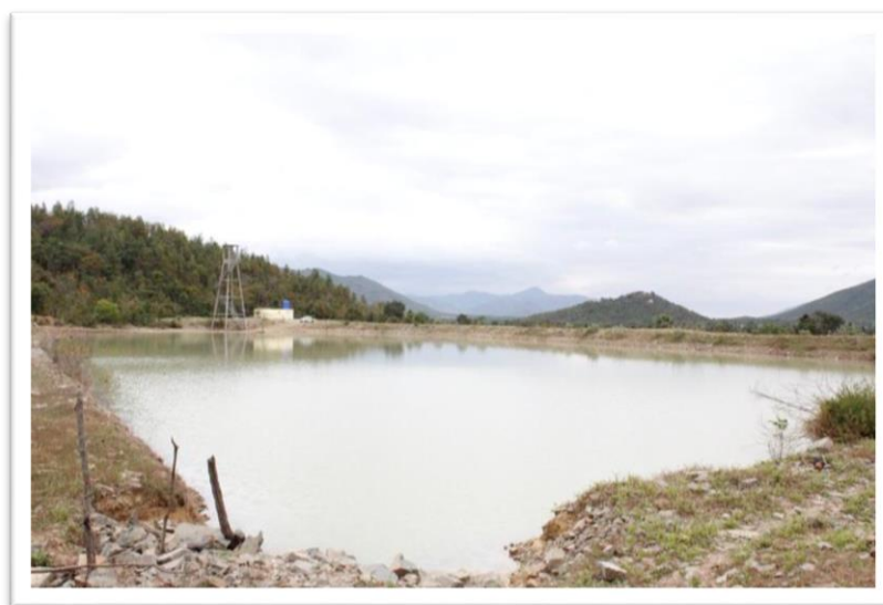
The renovated pond and water treatment plant
