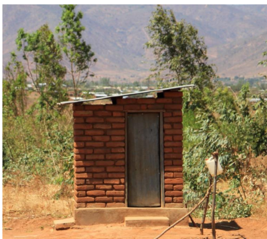
One of the new latrines with associated tippy-tap
