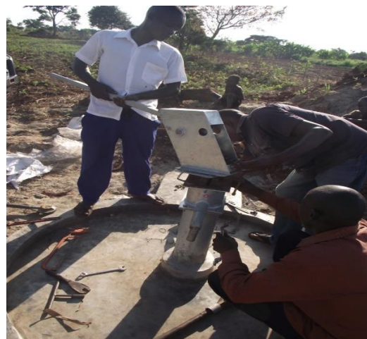
Installation of pump
