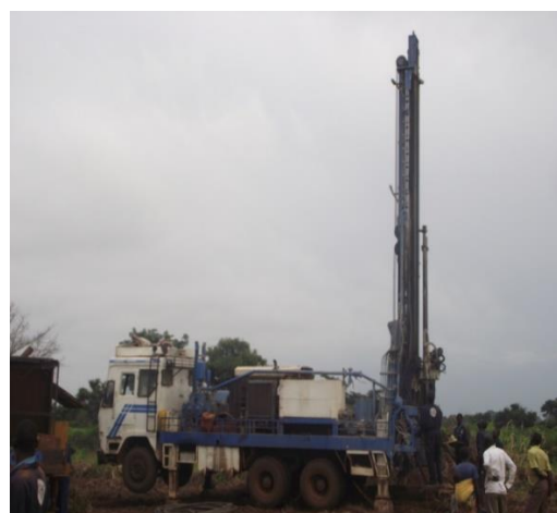
Drilling rig arrives on site
