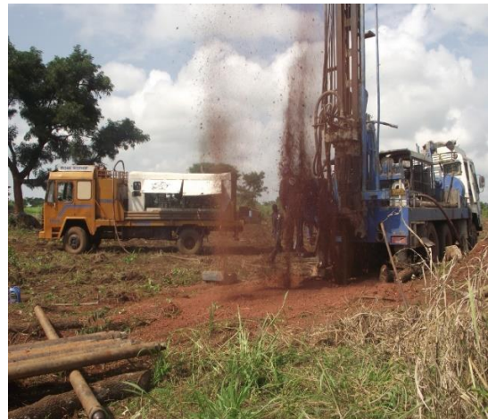
Drilling in progress
