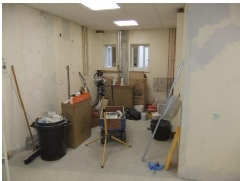
Kitchen area existing:
